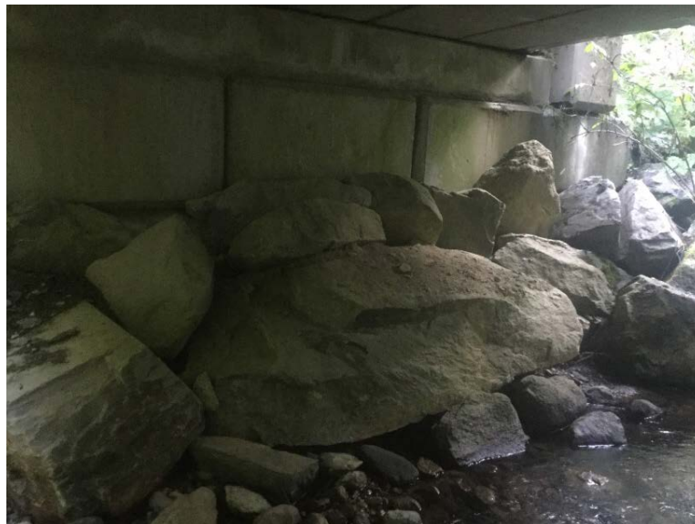
Left Bank Abutment when facing downstream
